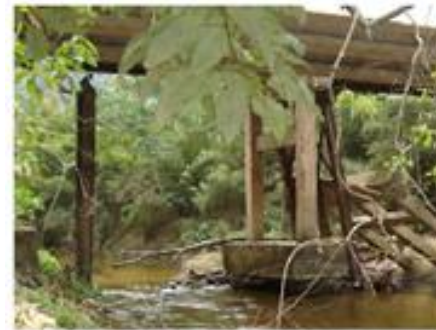
Bridge damage – debris flow after a flooding events in 2012 and March 2013 - Caragutatuba
