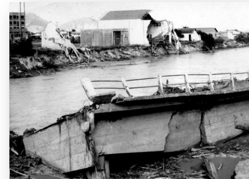
Bridge damage – debris flow after a flooding events in 2012 and March 2013 - Caragutatuba
